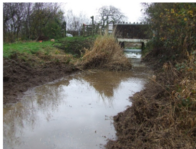
Exposed water after clearing vegetation
