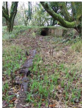
Remains of weir & overflow culvert.
